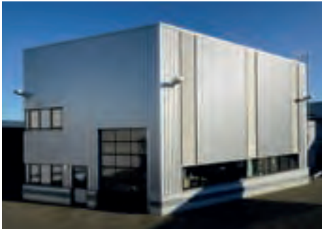
BOLL & KIRCH research centre including test laboratory
