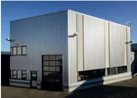
BOLL & KIRCH research centre including test laboratory
